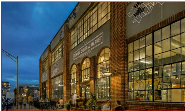
Opportunity to create an attractive frontage along the Market Hall edge which creates interest through the day and night
